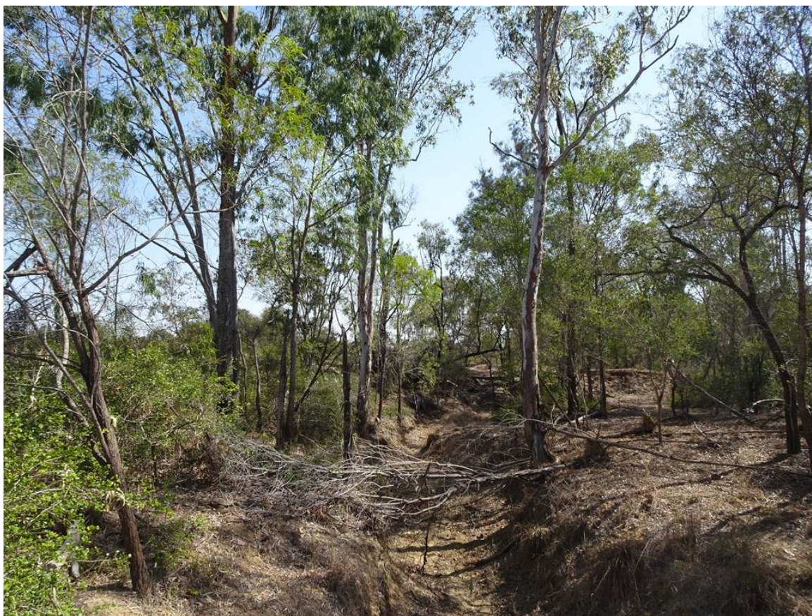
Above – Deeper incised channel and tree and shrub cover representative of the lower reach of Surveyor's Creek.
